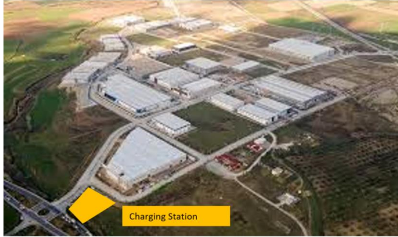
Figure 16: Electric Vehicle Charging Station Area
