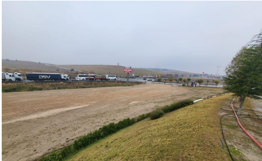
Figure 43: Fast Charging Station Area
